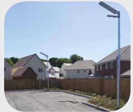
Right: Prolectric Street Lights
